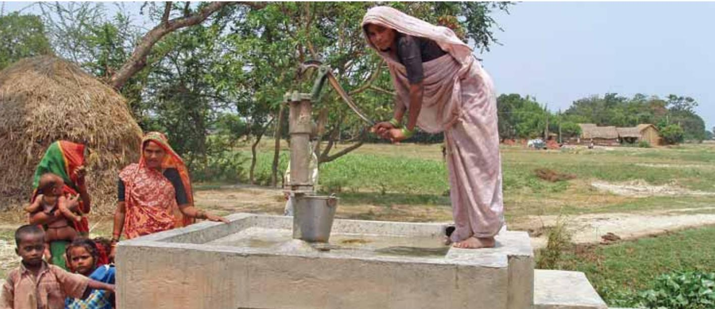
Villagers in Harhi, India, use their raised well, designed to withstand the regular flooding of the Ganges
